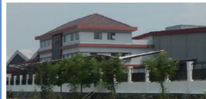
Full view of the plant
