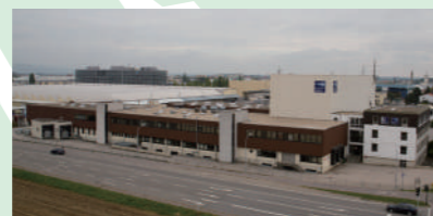
Full view of the plant
