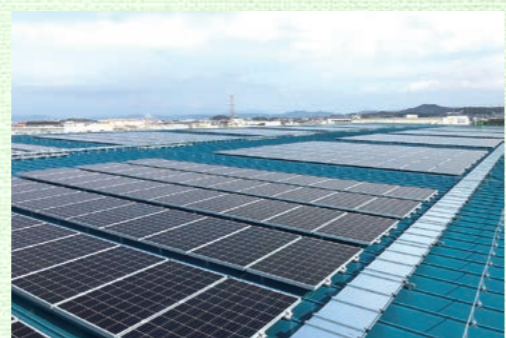
New factory building for plastic products of Nippon Closures' Komaki Plant
